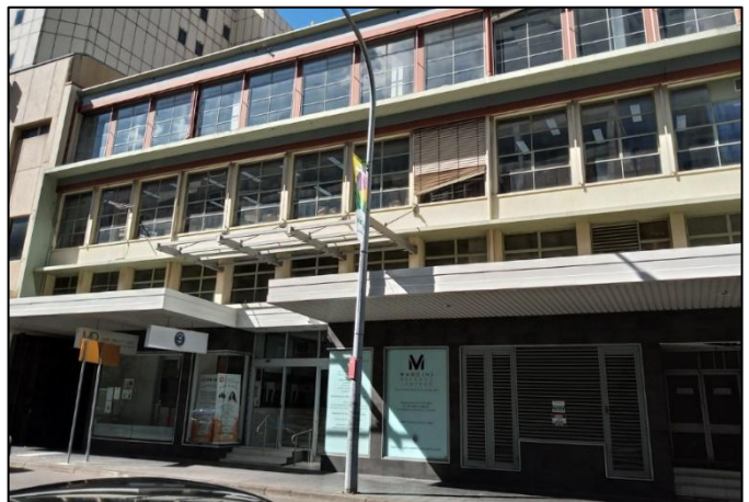
Figure 4: 89 Marsden St Parramatta (demolished per DA/802/2021)
